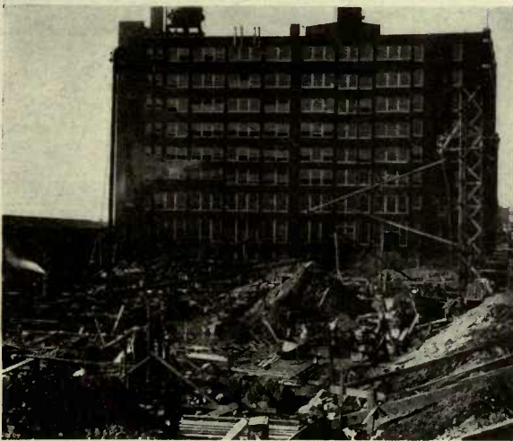
Ford Service Building, Long Island City, N. Y. Concrete Foundations and Floors Waterproofed with Truscon Waterproofing Paste, Concentrated
